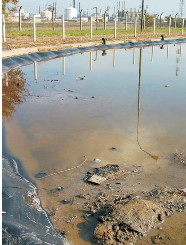
Temporary hazardous waste disposal site: lined lagoon, containing mainly waste from HIP PetroHemija Electrolysis plant
