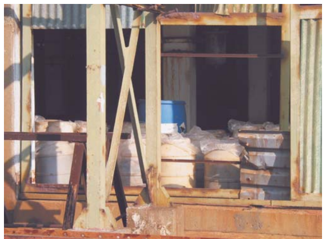
Temporary storage of drums with mercury-contaminated sludge, Electrolysis plant, HIP Petrohemija
