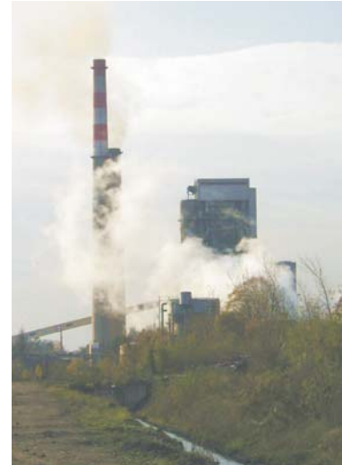
Stacks at power plant, Kolubara
