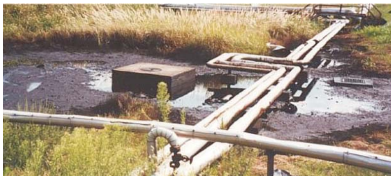
Bomb damage to oil pipeline at Novi Sad refinery, June 1999
