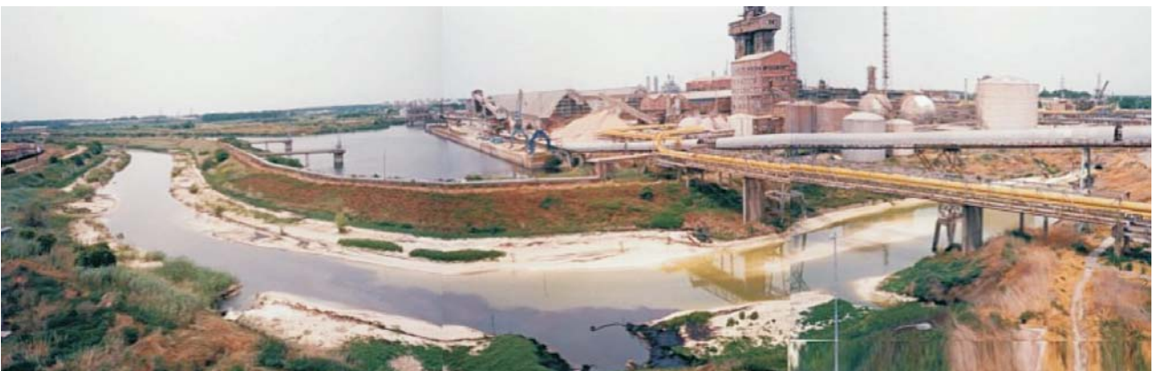
Pancevo wastewater canal, upstream part at the industrial complex, May 2002
