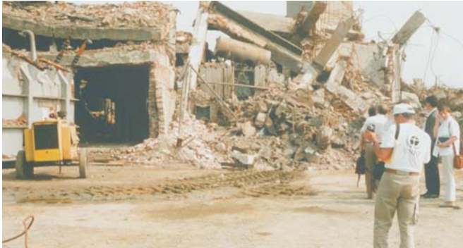
Transformer station (TS 3), destroyed by the bombing, June 1999
