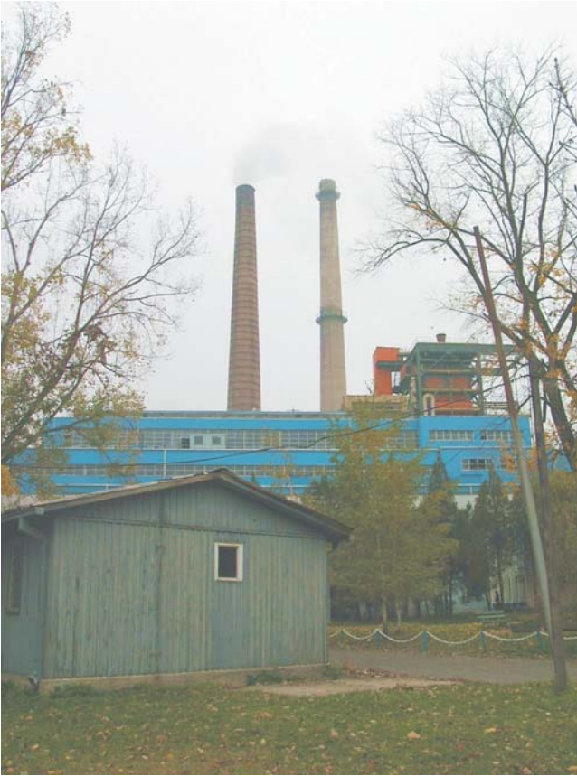
Stacks of power plant at Zastava, Kragujevac
