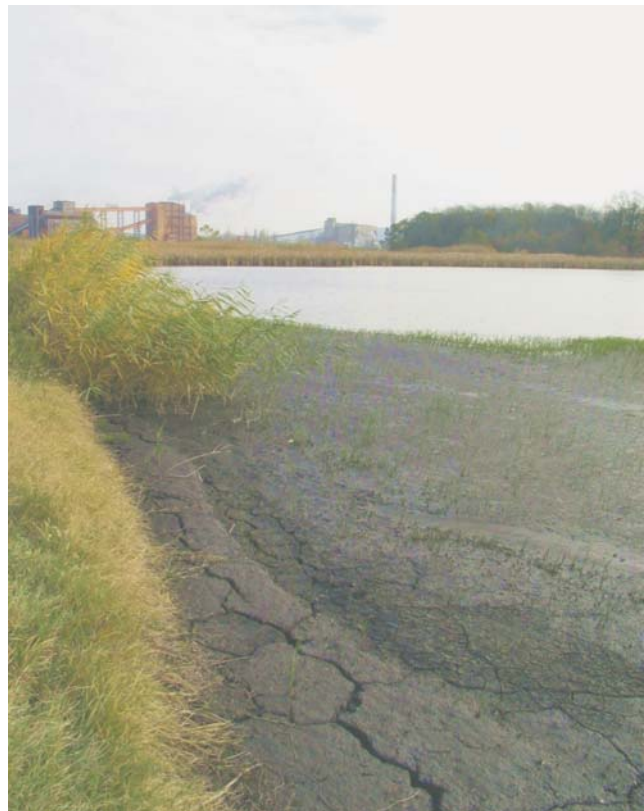
Wastewater settling pond, coal processing plant, Kolubara
