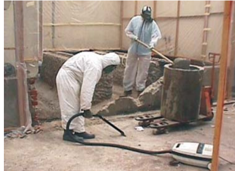
Clean-up works under protective tent at "Zastava Energetika" transformer station, September 2002
