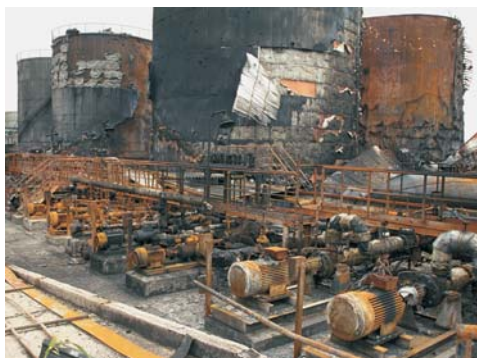
Bomb damage at NIS Oil Refinery Novi Sad, June 1999
