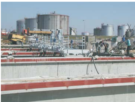
Concrete works and installation of equipment, August – October 2003
