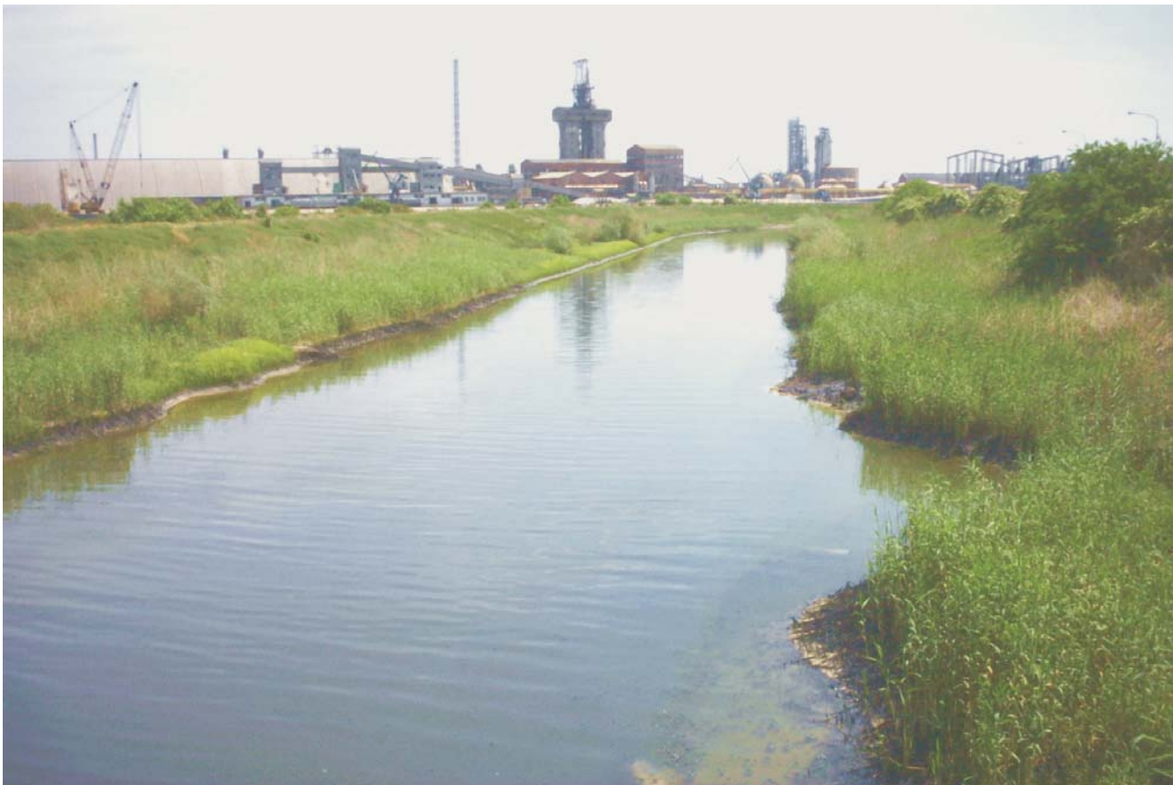
The wastewater canal and HIP Azotara, view upstream from the bridge at the middle of the canal
