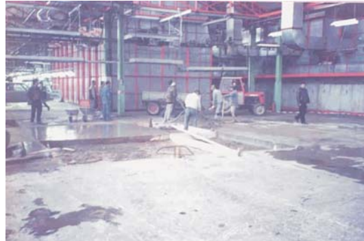
Covering of reclaimed area in paint hall with new concrete, March 2002
