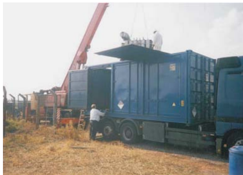
Packing of damaged PCB transformers at HIP Petrohemija, September 2002
