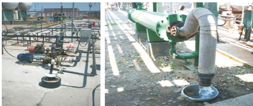
EDC Remediation - pumping of free-phase EDC and contaminated groundwater (left), discharge of treated water (right) at HIP PetroHemija Pancevo
