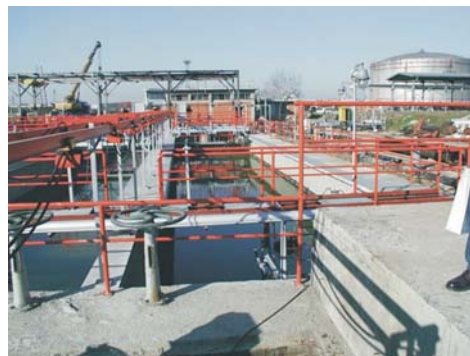
Rehabilitation of oil-separator completed, November 2003
