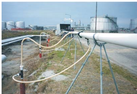
Remediation of free-phase oil on the groundwater table at Novi Sad refinery, January 2004
