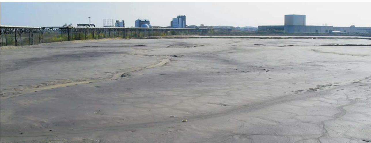
Storage of hazardous waste (jarosite) in an unlined landfill at Zorka complex, Sabac
