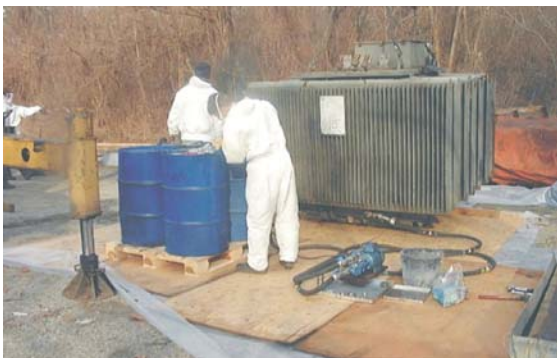
Re-packing of hazardous waste at UP-8 site, March 2002
