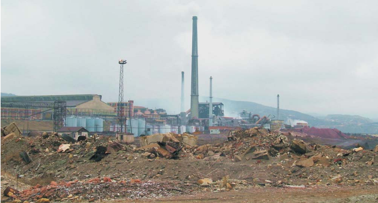
Air pollution sources at Copper Smelter , with industrial landfill (front), RTB Bor
