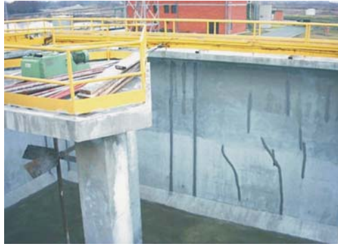
Trickling filter in operation, January 2004 (left). Repaired activated sludge basin interior (middle) and acid dosing pumps (right), January 2004
