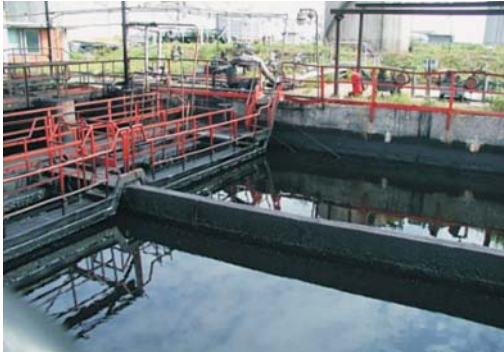
Pre-treatment facilities prior to rehabilitation, June 2002
