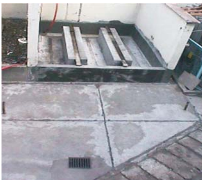
Transformer station site after removal of protective tent, September 2002
