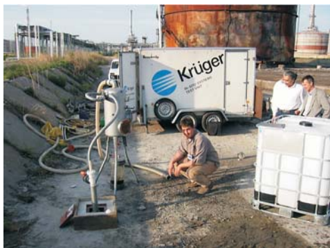
Novi Sad - Oil refinery: free phase remediation, pilot phase, May 2002
