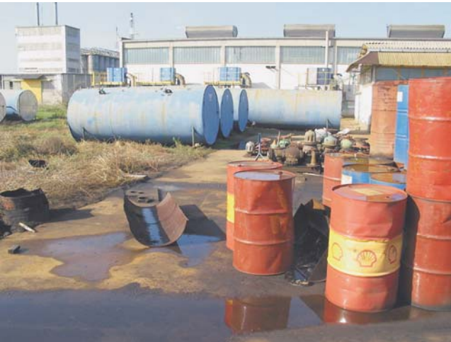
Outdoor storage of drums, Power plant, HIP Petrohemija
