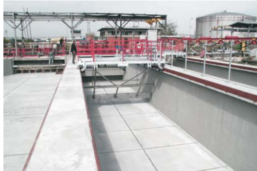
Concrete works and installation of equipment, August – October 2003
