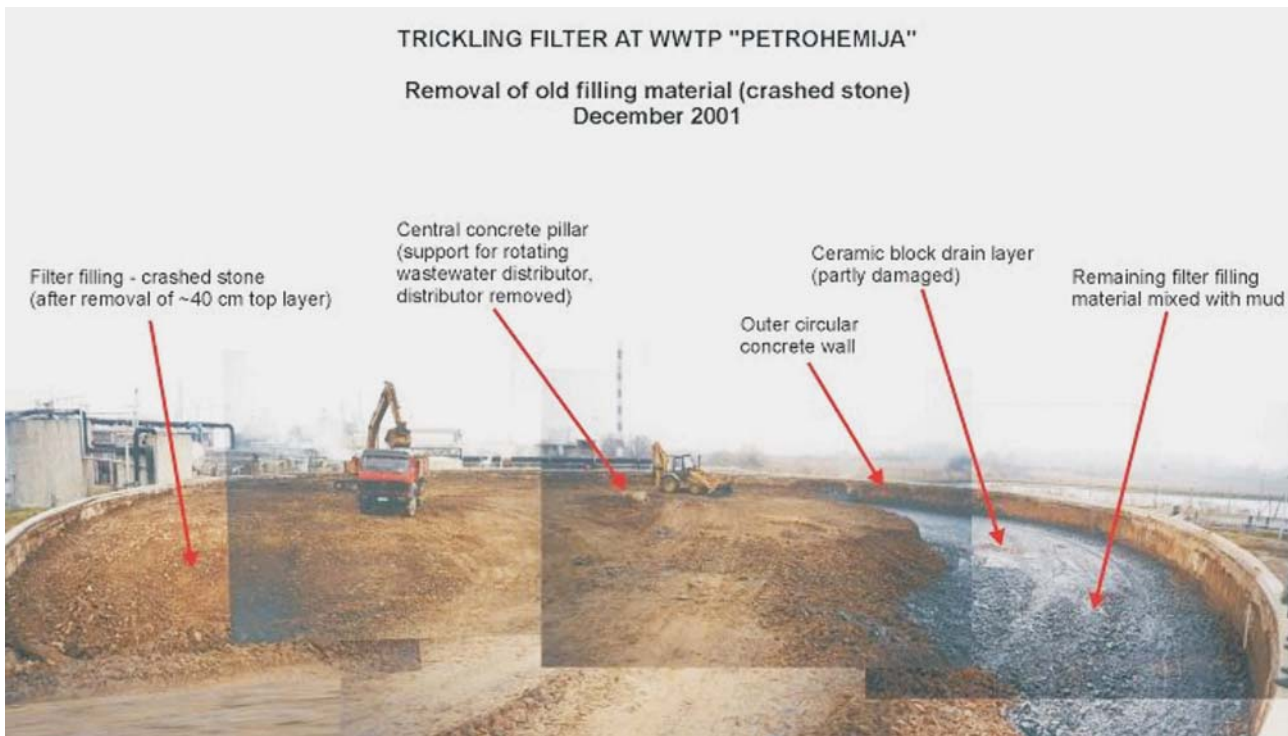
Rehabilitation of WWTP, trickling filter interior, at HIP Petrohemija December 2001
