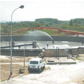
Rehabilitation of the WWTP trickling filter structure, June 2002 (left). Testing of new trickling filter equipment, December 2003 (right)
