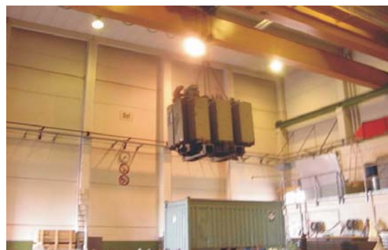
Unloading of damaged PCB-transformer at disposal facility, September 2002
