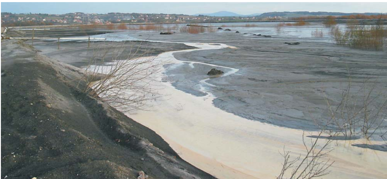
Fly ash disposal site, Kolubara power plant
